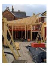
The timber frame and roof trusses arrived during November and the building is really starting to take shape. There is a long lead time for the windows, but the building will be made watertight to ensure the project can keep moving forward. The contractors are working hard to keep disruption to a minimum.
